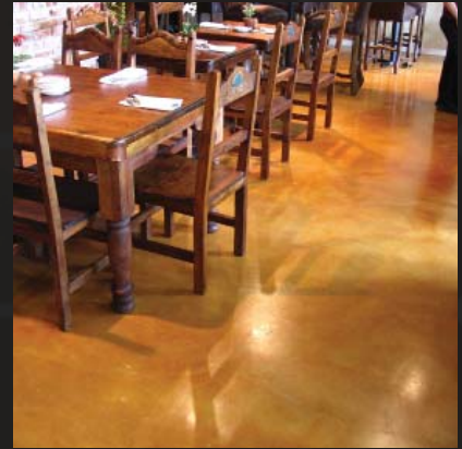
Interior Commercial Stained and Sealed Concrete Flooring
