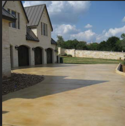
Exterior Stained and Sealed Concrete
