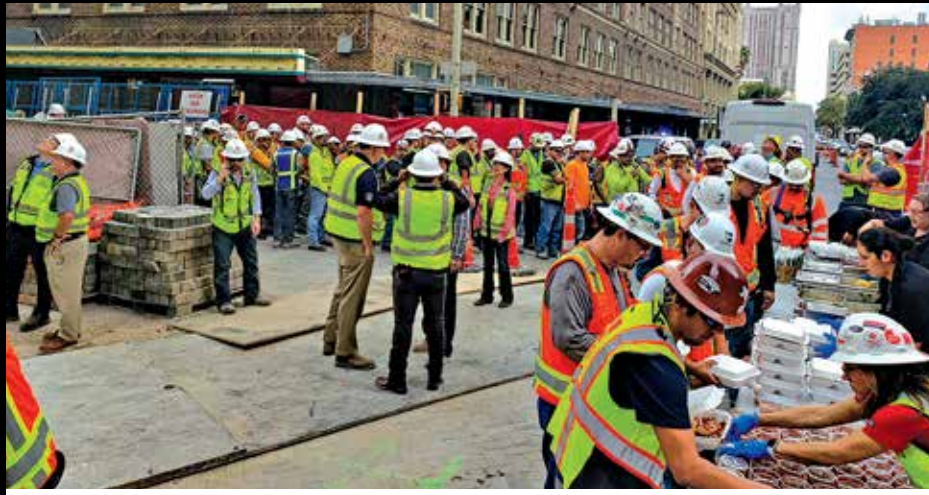
Sundt Construction Inc. celebrated the topping out of the Canopy by Hilton San Antonio Riverwalk at the northwest corner of N. St. Mary's and Commerce. The 22-story property will feature more than 3,000sf of meeting space, 195 guest rooms and a restaurant with an outdoor terrace overlooking the Riverwalk. Gensler is the architect of record for the project, which broke ground in 2017. The project is scheduled for completion in 2020. -cmw
