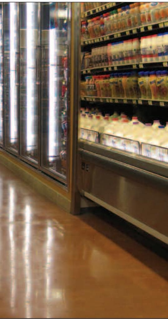
not provided integrally, acid stains or dyes may be used to color the concrete surface. As is the defining characteristic of polished concrete, there is no need for topical sealers or wax to cover and “lock in the color”. The achilles heel however of polished concrete floors are acids, which can etch the surface leaving the concrete susceptible to staining and uneven wear. Considerations should be made for any situation where mild or strong acids will be in contact with the flooring.
